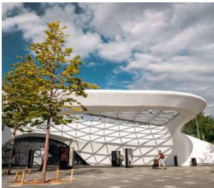
Figure 5. «Media Center» in Zaryadye Park, Moscow, Russia. Timur Bashkaev, Timur Bashkaev Architectural Bureau (ABTB), 2016-2017.
